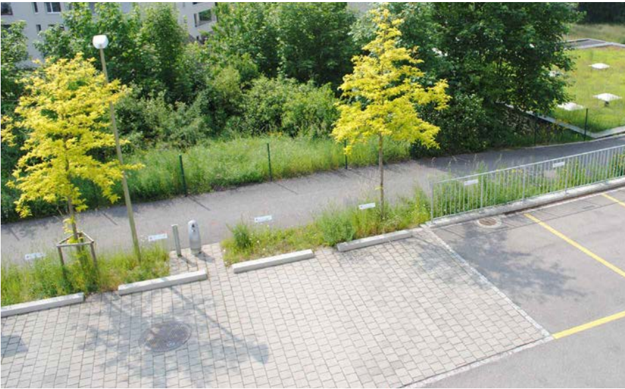
Use Green Infrastructure and Low Impact Development (LID) principles to treat runoff from surface parking lots.
