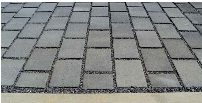
Permeable paving systems allow water to pass around pavers and infiltrate into the soil, reducing runoff and filtering stormwater.
