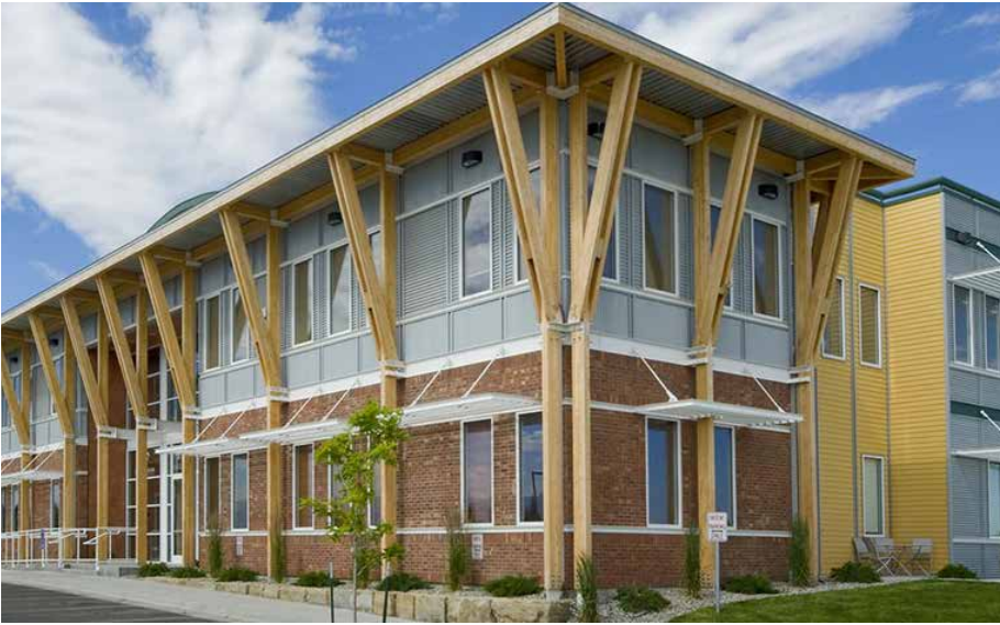
Integrate architectural details with facade articulation. Use a combination of elements such as exposed posts, beams, trusses and brackets.
