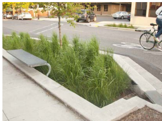
Bioretention areas or rain gardens are planted areas with subsurface materials that store and filter stormwater while supporting vegetation
