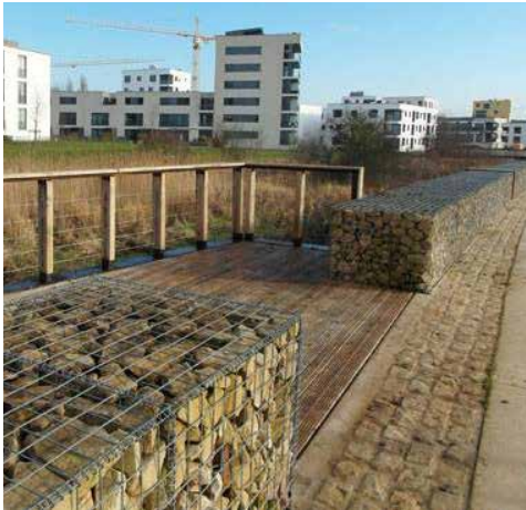
Fences and walls should be used for areas that need to completely exclude pedestrian access.
