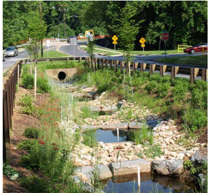
Open swale conveyance channels allow water to move across the site in a natural setting that increases water infiltration.
