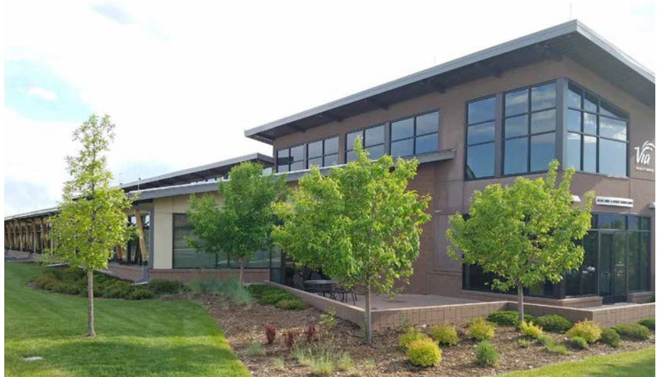
Ground floor wall offsets provide relief at the pedestrian level to avoid a long uninterrupted wall.
