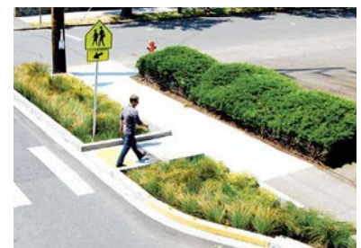
Infiltration planters are bioretention areas with deeper above ground containers to allow water to sit and slowly infiltrate
