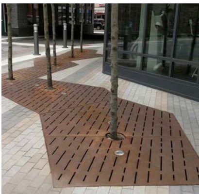
Tree trench filters are tree planting areas, often covered with a grate, that include large underground areas with materials that store and filter stormwater
