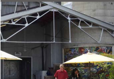
Details can provide a sense of human scale to a building.
